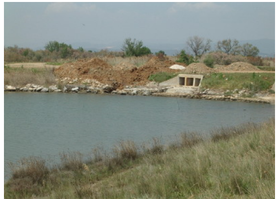
Hydraulic works in the delta.
