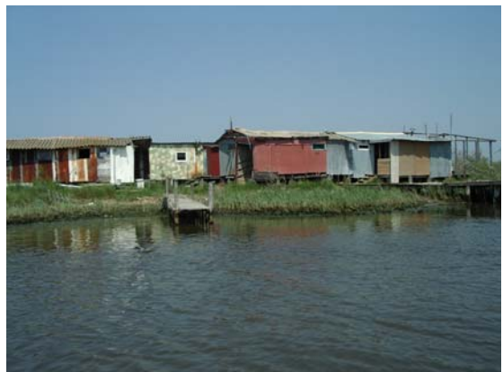
Illegal huts within the Ramsar wetland.
